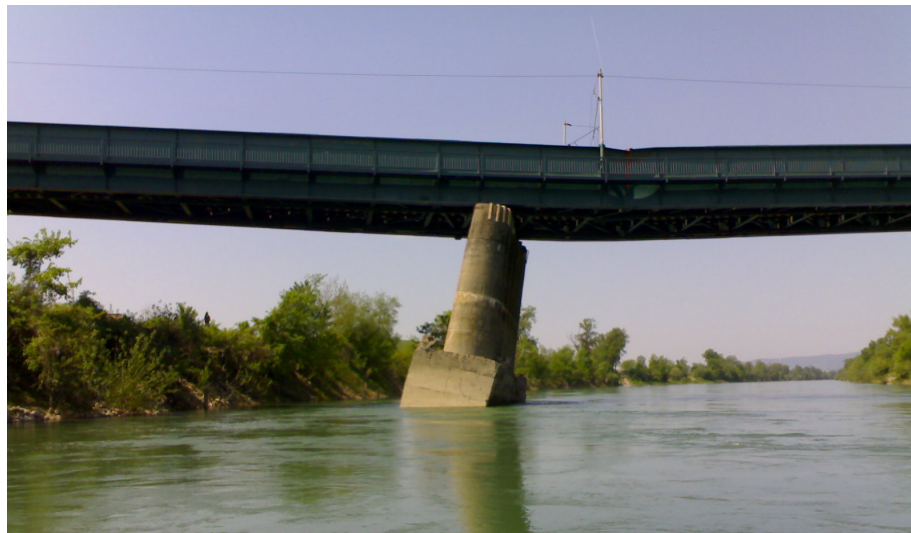
Figure 43: The railway bridge Jakuševac in Mičevac on the Sava River that collapsed on March 30, 2009, at 22:30 when a freight train was crossing the bridge, the bearing structure of the bridge lost its stability and resulted in a deformation of the bridge structure and tracks
