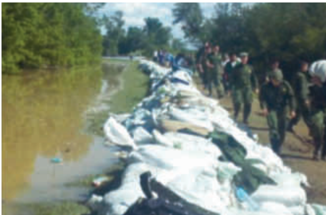
Emergency measures along a low part of the dike upstream of Šabac, Serbia
