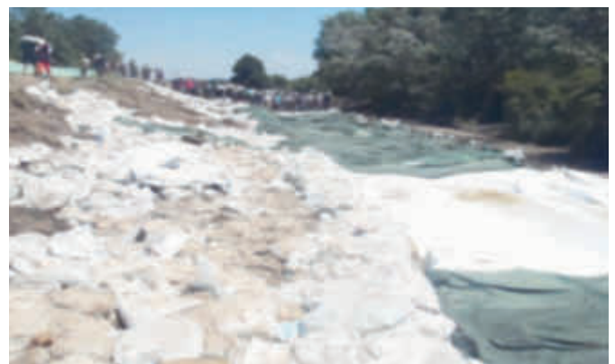
Emergency measures along a part of the dike where reconstruction was ongoing, upstream of Šabac, Serbia
