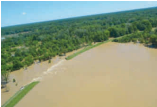
Dike breach in Kopanice, B&H
