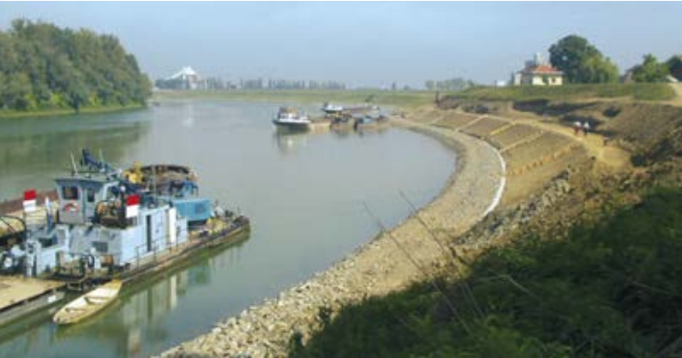
Figure 4 ► Sloping revetment built of broken stone
